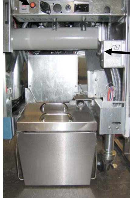
Melting unit power switch
